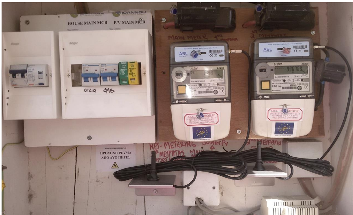
Figure 8 Double meter installation with import – export and generation meters
